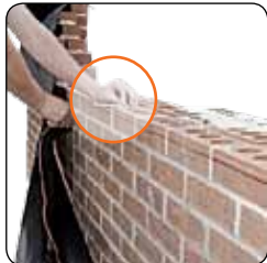
Line Pin being used for aligning wall with corner
